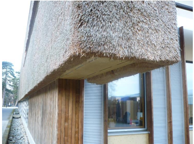
Exterior walls made of locally sourced thatch
