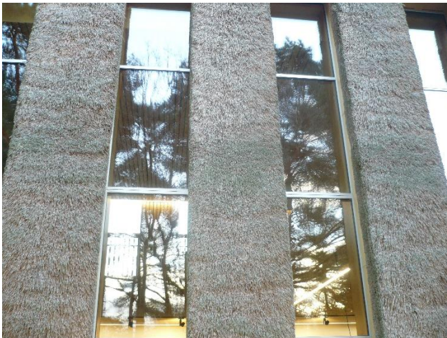
Exterior thatch walls are expected to have a lifespan of 50-60 years before replacement
