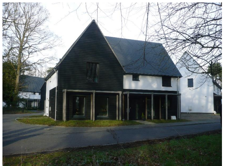
Material pallet of white render, black stained timber cladding & slate/plain red roof tiles reflects materials used in adjacent Carrowbreck House
