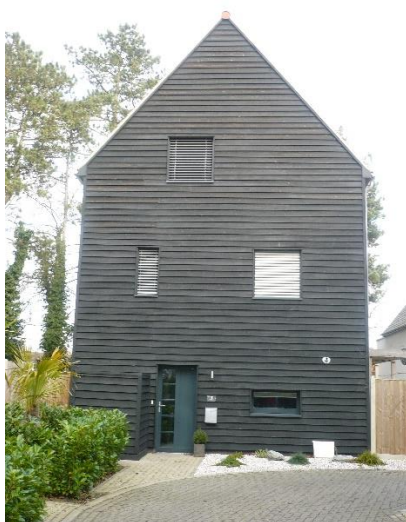
Material pallet of white render, black stained timber cladding & slate/plain red roof tiles reflects materials used in adjacent Carrowbreck House
