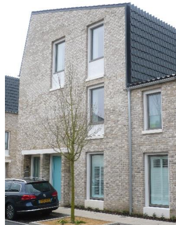
Landmark buildings 'bookend' each terrace and roofs oriented for maximum passive solar gain
