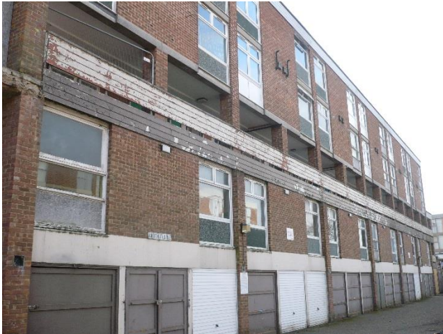
Remaining street frontages dominated by garages
