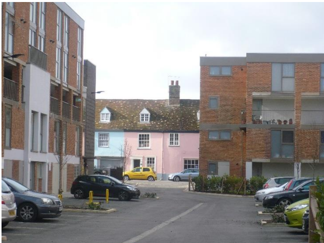
'Selective demolition' of key areas of estate to reveal surrounding context
