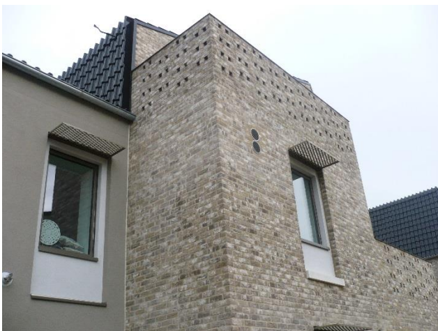
Careful detailing of window reveals and external brickwork
